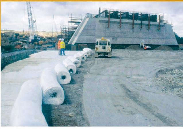
$Tensar\ Basetex\ in\ a\ Tensioned\ Membrane\ Load\ Transfer\ Platform\ supporting\ an\ embankment\ for\ high\ speed\ railway.$
