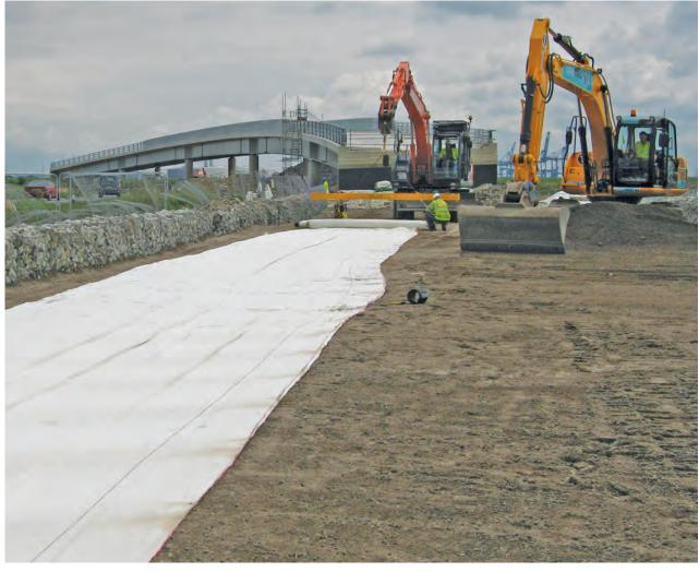
$In stall at ion of \textit{Basetex in a Tensioned Membrane Load Transfer Platform over bored piles on the \textit{A228 highway embankment over all uvium in Kent.} \\$
