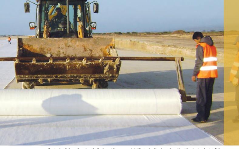
Basetex installation at Oran airport in Algeria providing permanent stability to a load bearing surface with rapid and cost saving installation.
