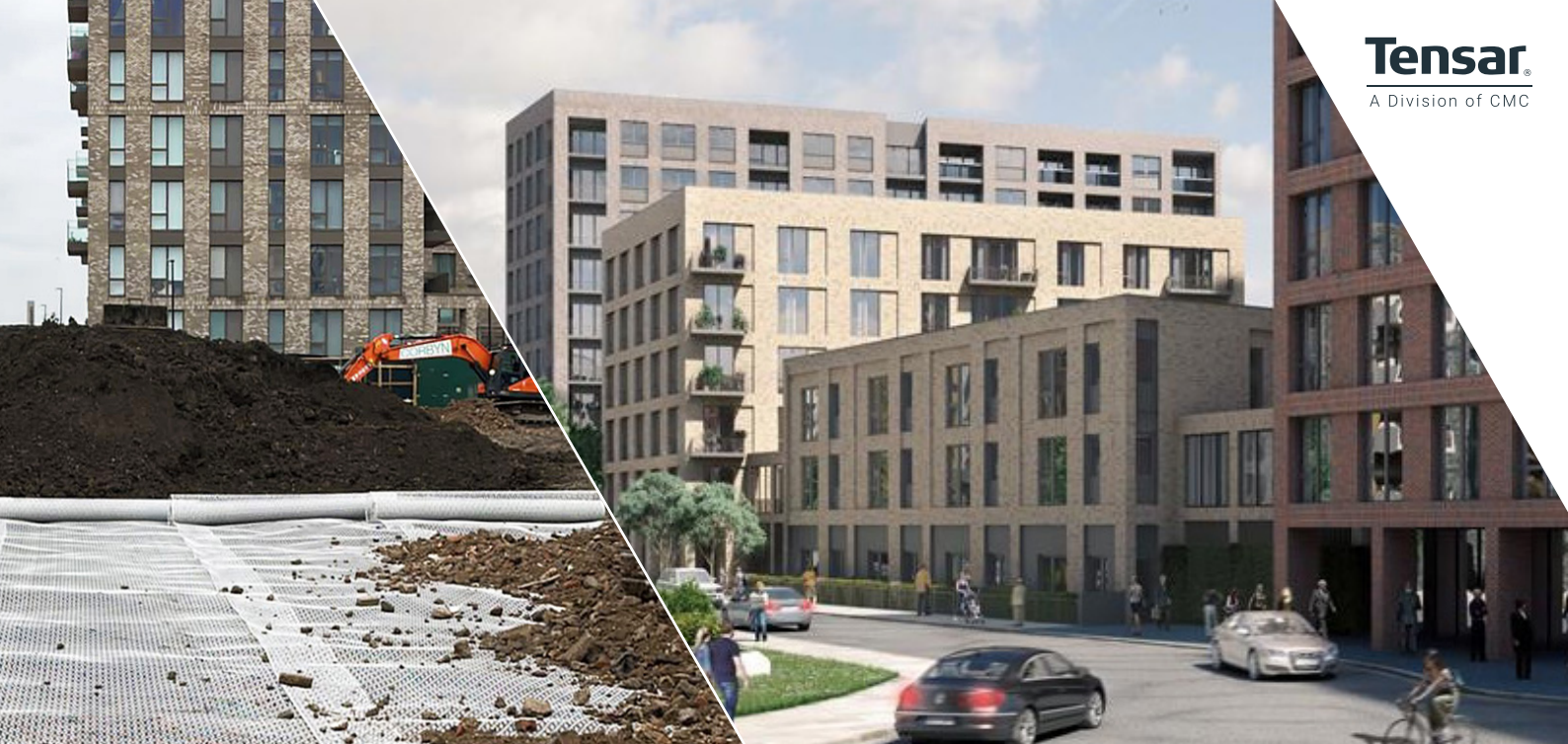
CGI of the Gallions - Phase 3b development. Tensor InterAx geogrid (inset) installed below the piling mat enabled a massive reduction in fill volume
